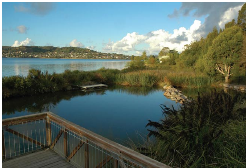
This wetland at Lake Macquarie was built by the Office of the Lake Macquarie and Catchment Coordinator to filter stormwater run-off into the lake, and is an example of a successful collaboration between agencies, councils and CMAs. (Photo: Nicholas Shields)
